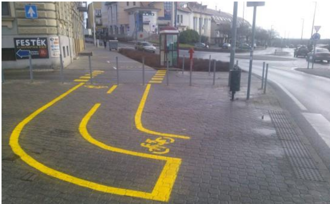
Figure 21: Bicycle road in the centre of Pécs, in Alsóhavi Road
